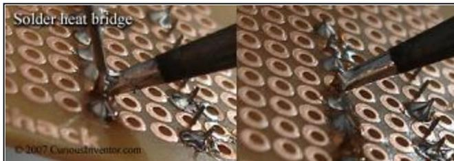
If there isn't enough solder on the iron tip from "tinning the tip," little heat will transfer from it (a "dry" tip). It's important to have a little solder between the iron tip and work. This is called a "heat bridge." Melt a small amount of solder between the tip and lead, and then continue adding solder on the opposite side.
